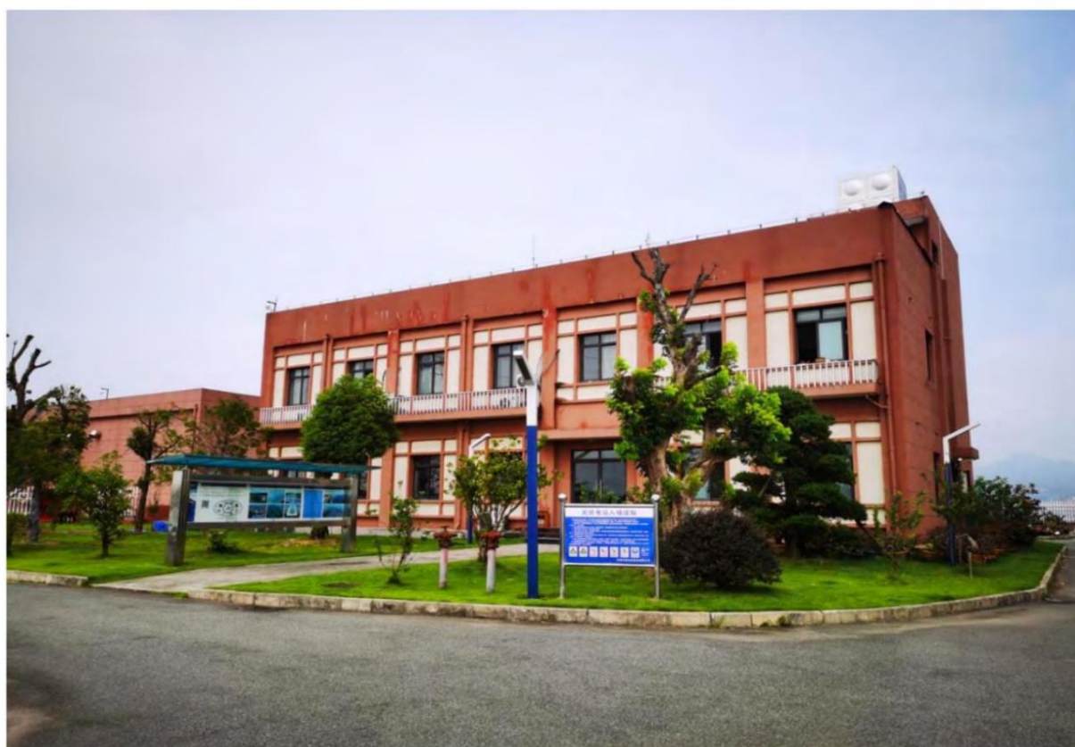
Figure 10 Greening in the booster station
