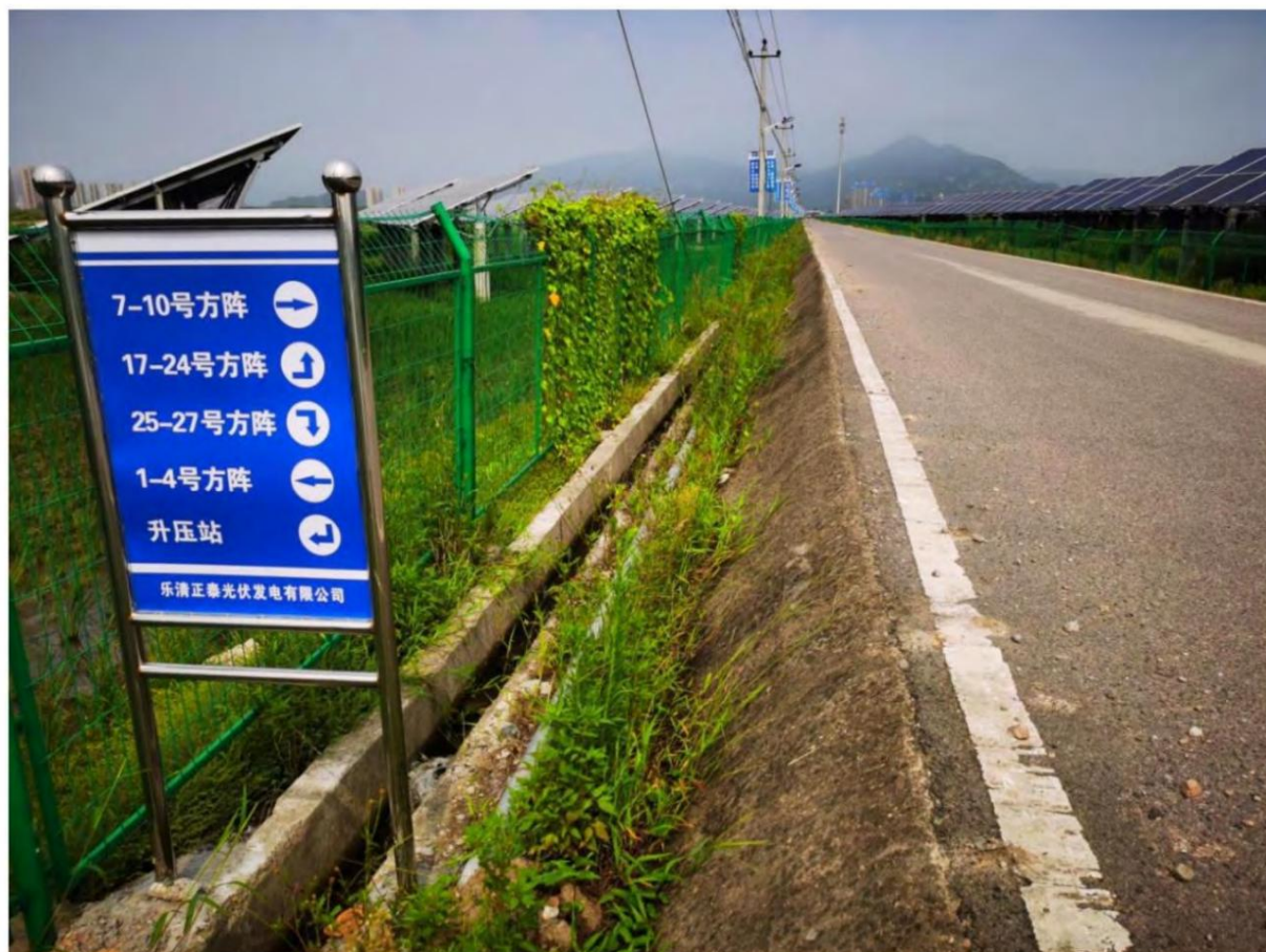
Figure 7 Drainage ditches on both sides of the road
