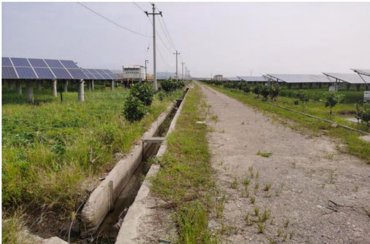
Figure 6 Drainage ditches on both sides of the road
